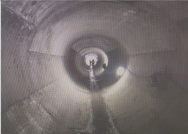
Newly installed outlet pipe lining Photo courtesy of NorthWestern Energy
